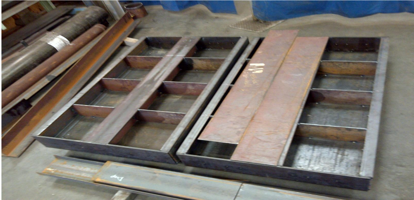
Fabrication started on new 159 weir. Expected completion for installation this winter.
